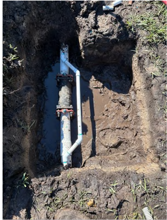
Mainline repair along Ayersworth
