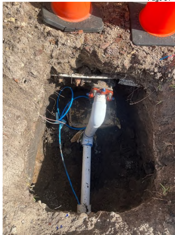
Mainline repair on north side of Clyne Field
